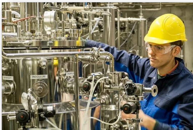
Working on the biomass pre-treatment Pilot Line
