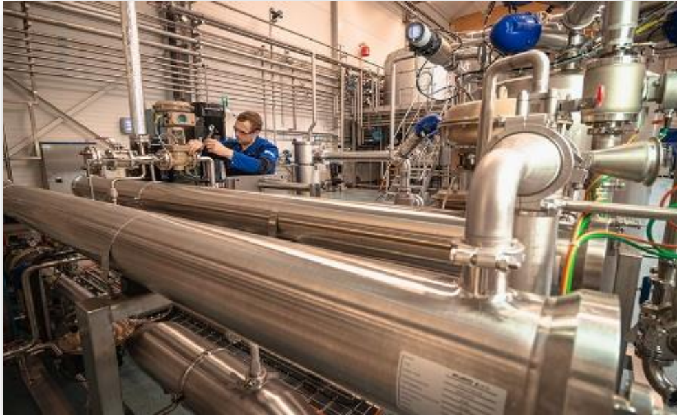
PL6 located at the Bio Base Europe Pilot Plant
